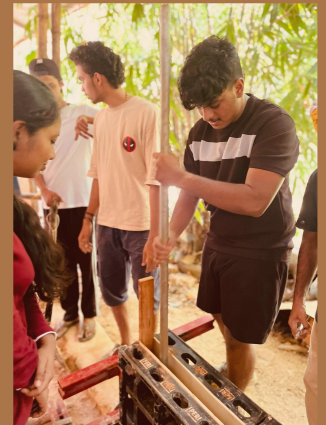
Compact process involved in rammed earth
