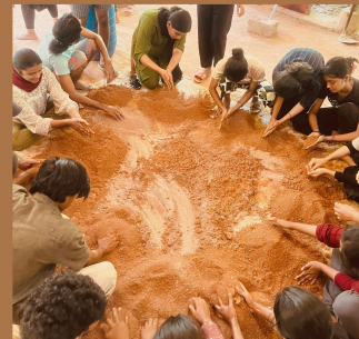
Mixing lime and sand for rammed earth
