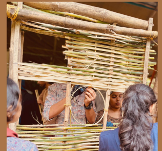
Wattle construction using bamboo
